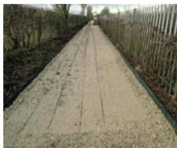
All-in-one surface forming drainage edges
