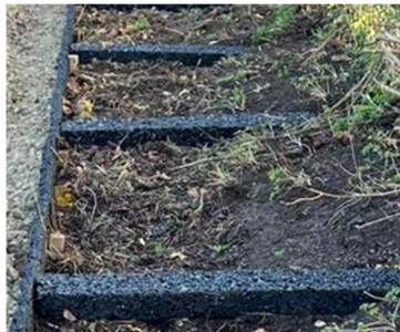
Combined drainage edges and drainage spurs
