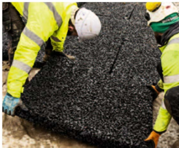
Modular drainage layers deliver Avg. 45% void space
