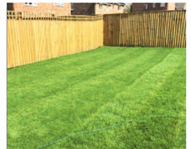
Hydrotrench® drainage system – after installation
