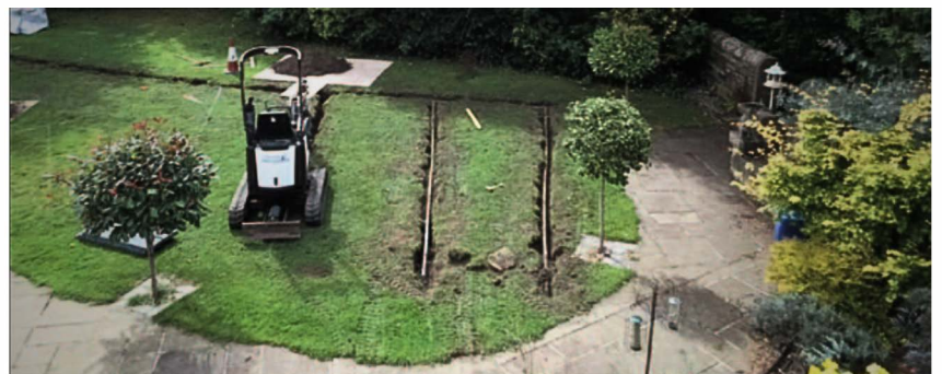
Hydrotrench® sustainable drainage system garden installation with reduced excavation
