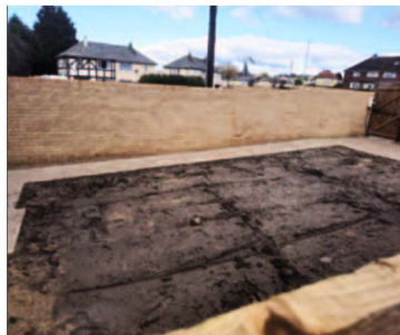
Hydrotrench® drainage system – after installation
