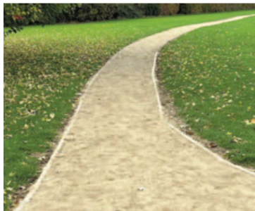
Path with integrated sustainable drainage
