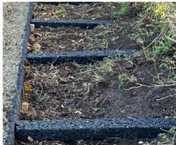
Combined drainage edges and drainage spurs
