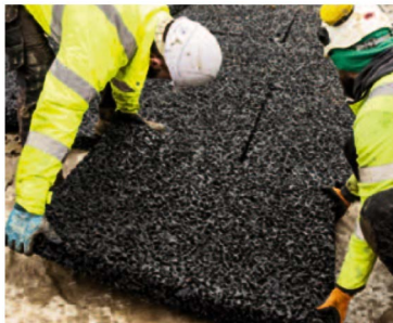
Modular drainage layers deliver Avg. 45% void space
