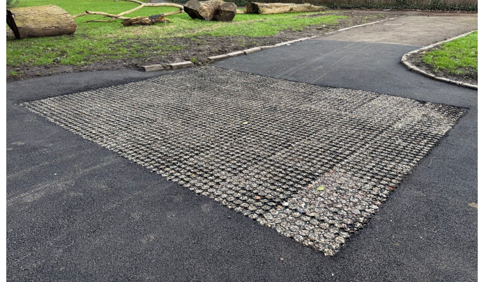
After: accessible, drained route
