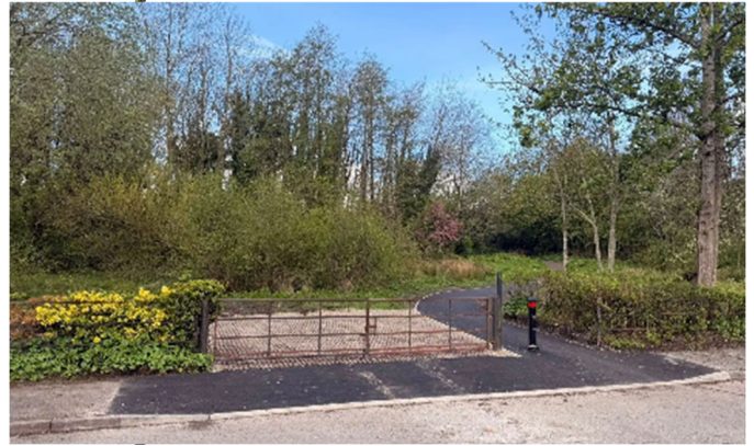
After: accessible, drained route
