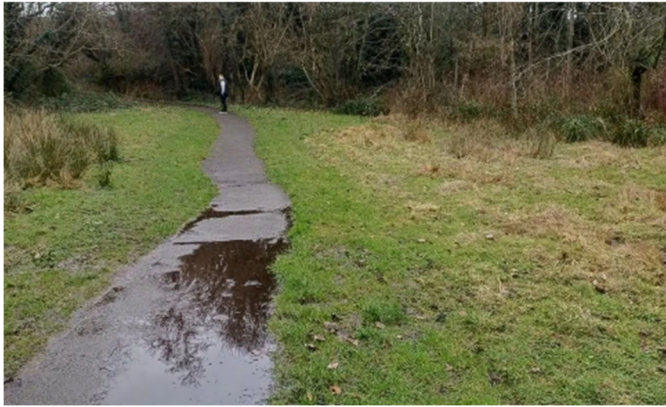
Before: waterlogged conditions
